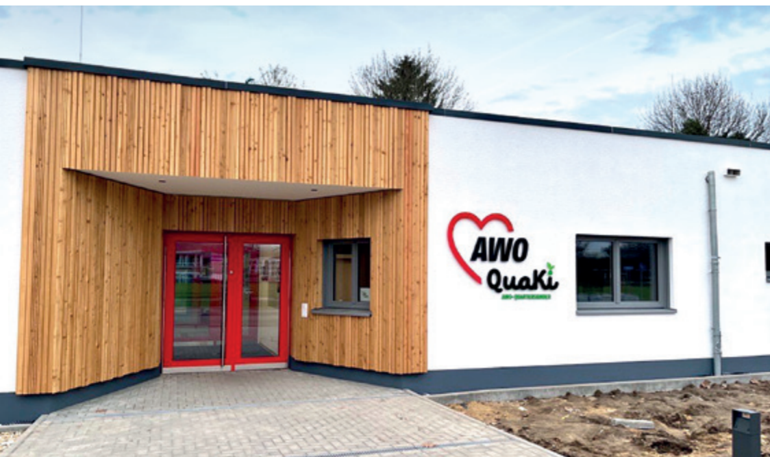
QuaKi is the local kindergarten in Monforts Quartier in Mönchengladbach. Our contribution to company childcare in a sustainable setting.
